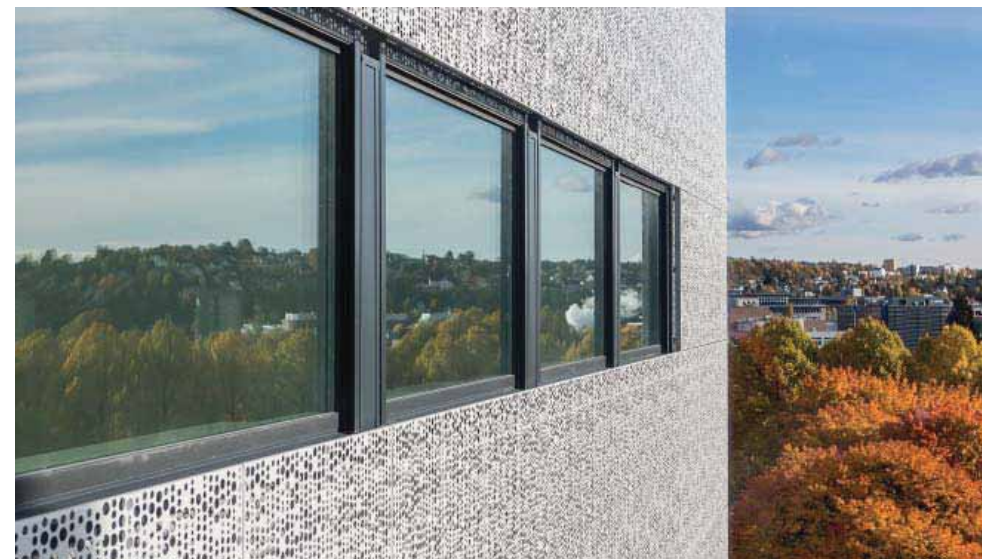
▲ The new perforated aluminium façade is part of the new energy efficient building envelope and creates a bright entity in the cityscape [Tove Lauluten].
