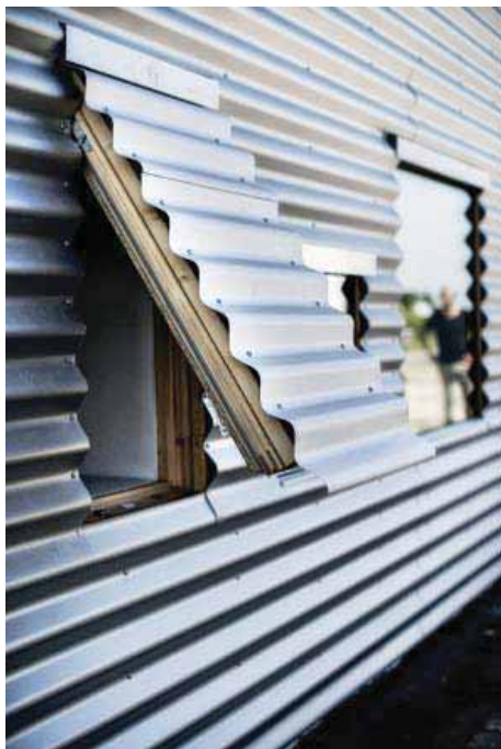
▲ Ventilation shutter and fixed windows [Polfoto].
