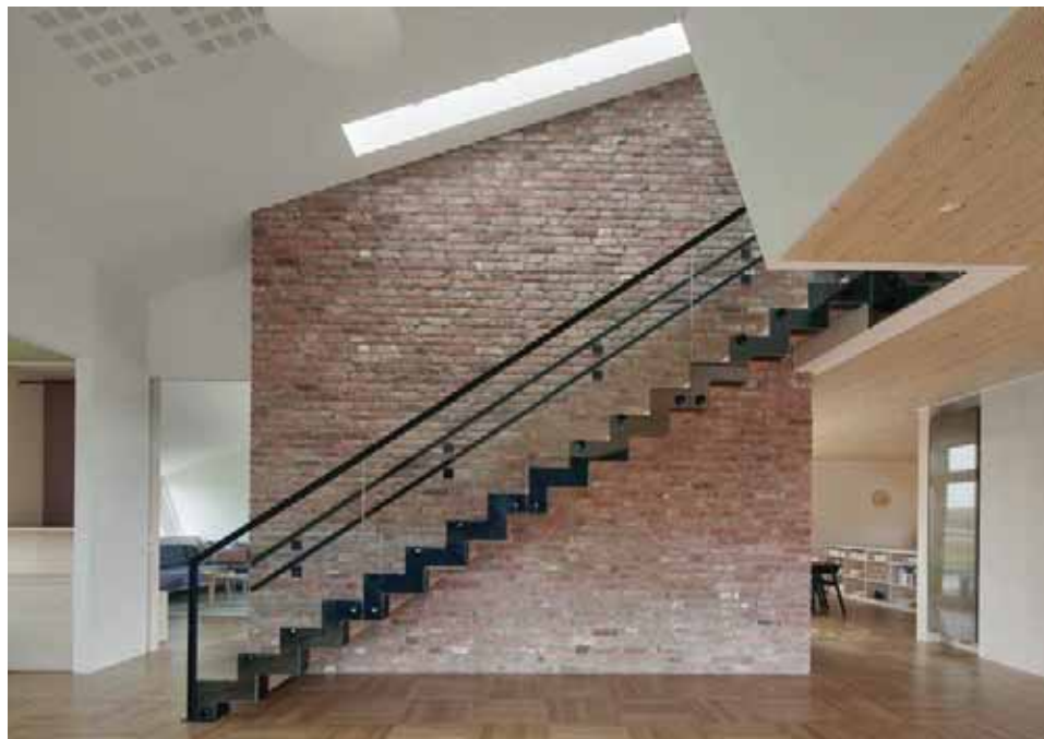
▲ The wall of recycled brick not only takes effect as passive energy storage but also highlights the sculptural staircase [Bruce Damonte].
