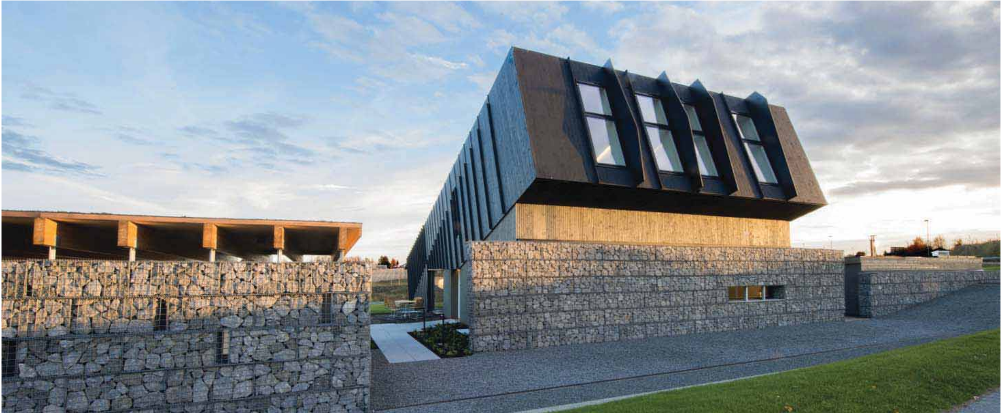
▲ Large fins protect the bedroom windows from solar heat [Paal-André Schwital].
