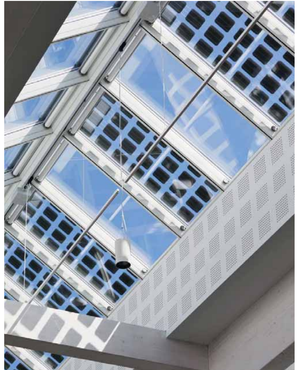
▲ Energy production and sun shading in one [Laura Stamer].
